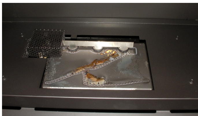
Figure 31e. Completed Placement of Rock Guard.
