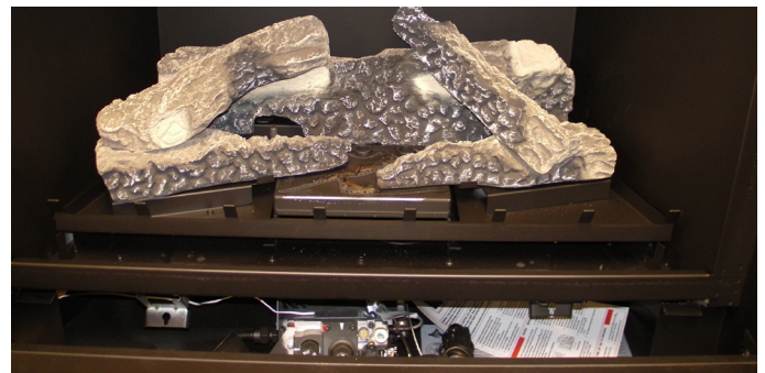
Figure 31a. Firebox with logs prior to ceramic fibre rock installation.
