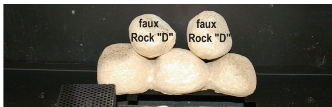
Figure 32e. Place the remaining (2) two faux "D" ceramic Rocks on top of faux the "A" (3 in 1 ceramic rock.) (flat surfaces of rock against back of firebox).
