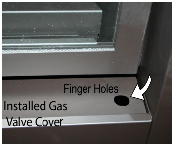
Figure 26. Removing and installing the Horizontal Access Panel
