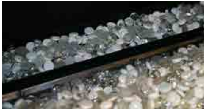
Figure 25. Completed firestone installation. Second Gen burner shown.
