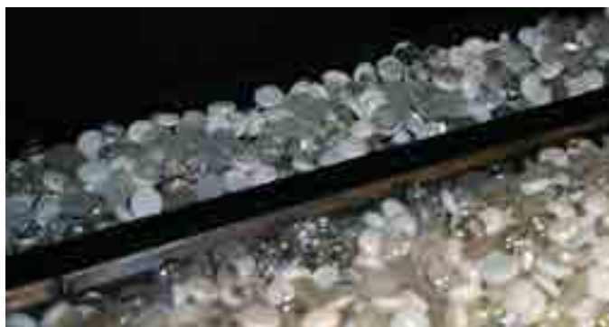
Figure 28. Completed firestone installation. Second Gen burner shown.
