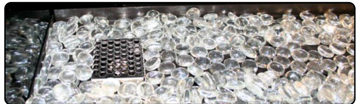
Figure 24.b Completed firestone installation
