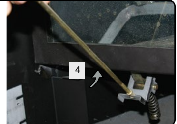
Figure 23.g Lift the door up and out of the fireplace frame
