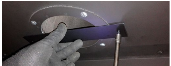
Figure 8.b.c Restrictor plate Installation
