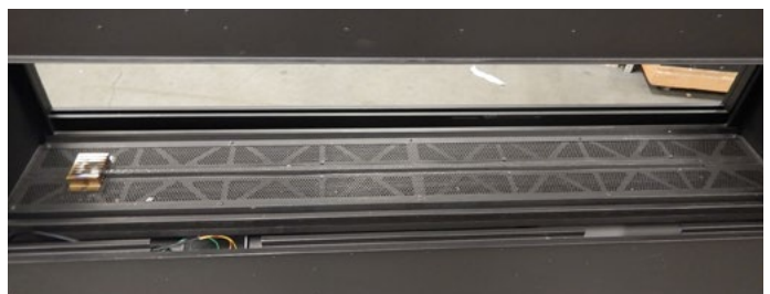
Figure 25.g Insert pilot cover/door/screen
