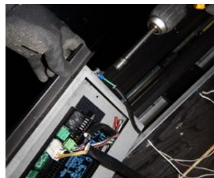
Figure 24.b Remove existing basic board
