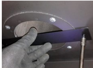
Figure 8.b.c Restrictor plate Installation
