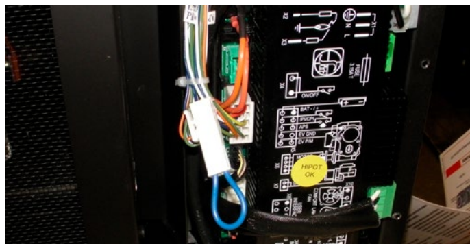
Figure 19.c Connectez le câble de raccordement CPI
