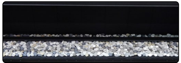
Figure 11.f Completed Speckled Stone installation
