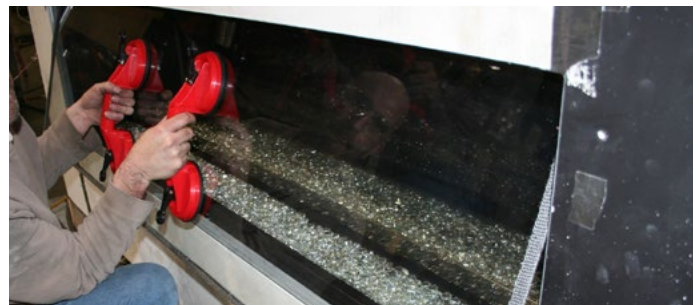
Figure 11.c Window Removal (using glass lifting tools).
