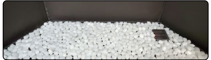
Figure 24.bb Completed firestone installation
