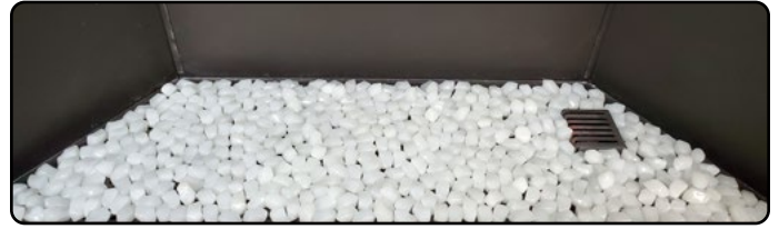
Figure 24.bb Completed firestone installation
