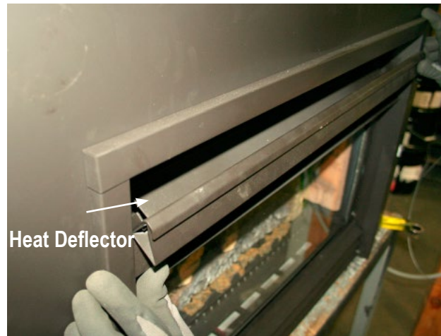
Figure 9b. Installing the upper louvres.
