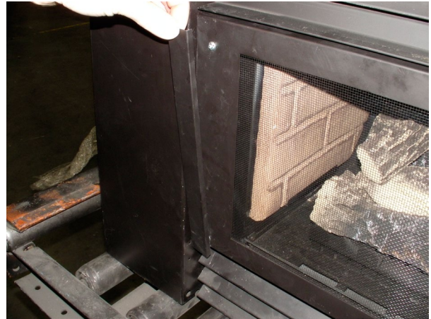
Figure 11a. Removing the screw covers.
