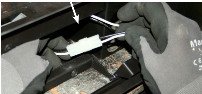
Figure 10b. Connect Fan Speed Control wires.
