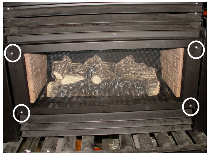
Figure 11b. Removing the screws.
