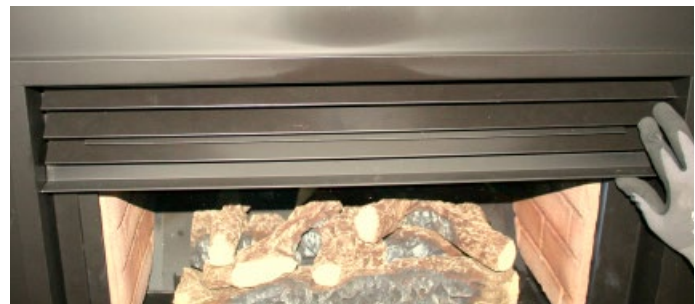
Figure 9c. Completed installation of Upper louvres.
