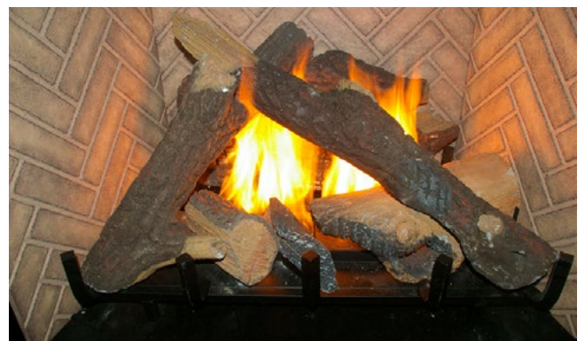
Figure 18m. Completed Log Set Installation.
