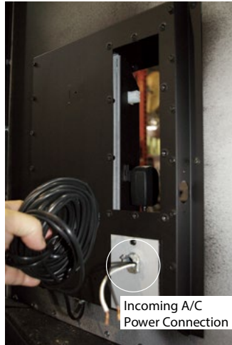
Figure 12. Incoming A/C Power , (connect per. Local Codes).
