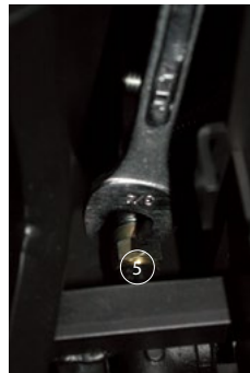
Figure 20d. (Loosening Gas fitting on burner).
