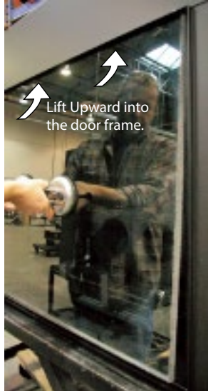
Figure 17. (Lift the door upward)
