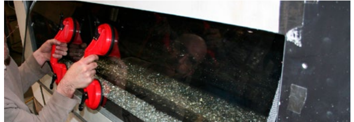
Figure 11.c Window Removal (using glass lifting tools).
