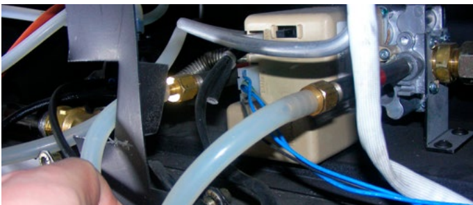
Figure 9.b Pressure testing
