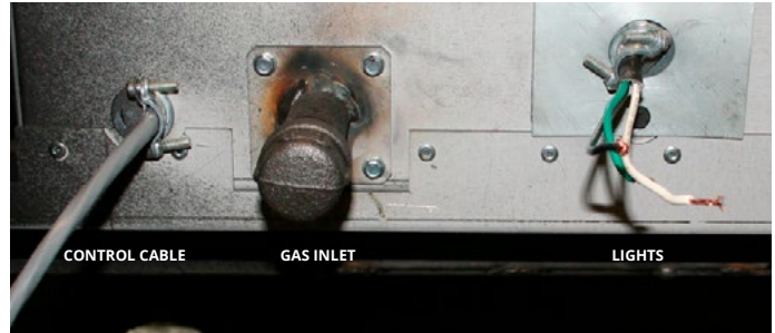
Figure 9.b.b Identifying the Gas Inlet
