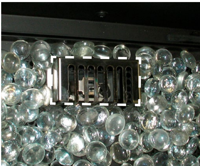
Figure 61. Do not place any media on top of the pilot shield.
