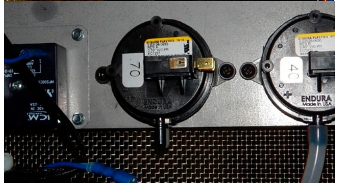
Figure 117. Disconnect grey wire.
