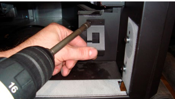
Figure 13 Attach switch bracket to front of fireplace
