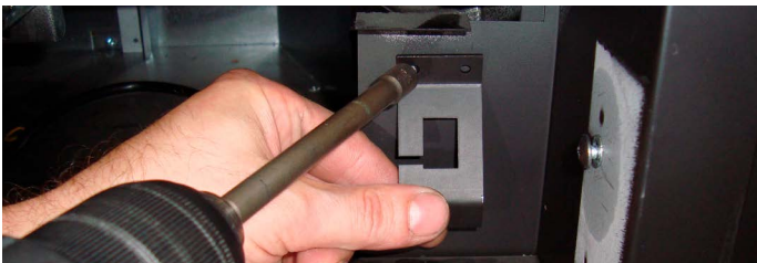
Figure 19 Attach switch bracket to front of fireplace
